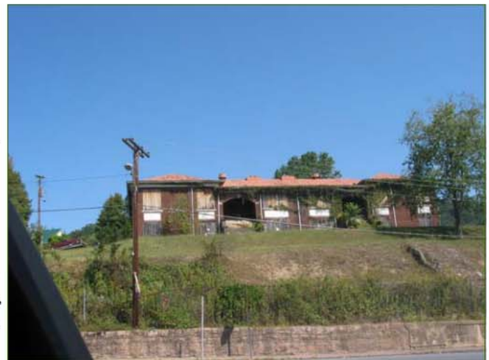
View of vacant Ansted High School Building. Redevelopment plans by the Town of Ansted include town offices, community center, and a small business center complex
