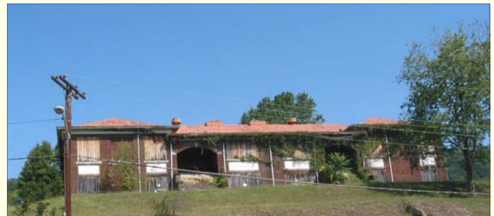
Above : Current View of Former Ansted High School
