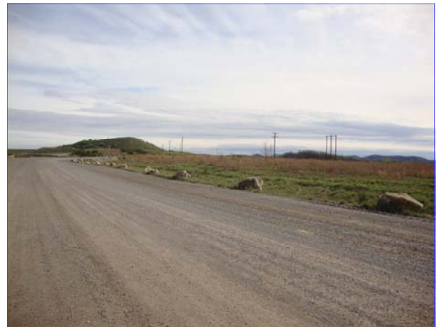
Arch Coal Birch River Surface Mine Complex near Cowen has an extensive road network, large sections of flat reclaimed land, and electric and water utilities
