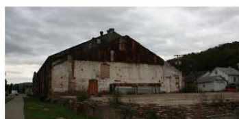
Former Brooke Glass Factory and adjacent Yankee Rail Trail
