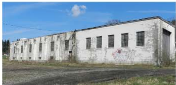
Potential rail trail in front of the Kern Valley Railroad Maintenance Facility
