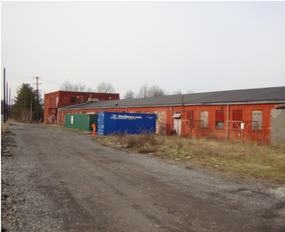
Above photo showing rear of Corbins building, which will be “deconstructed” to salvage structural materials.
