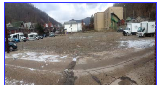
With Demolition Complete, the Site is Now Ready for New Development
