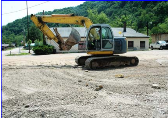
Completion of Petroleum Impacted Soil removal at DOH Garage (May 2011)
