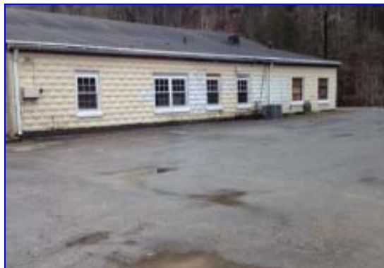
Exterior of “New” BDA Offices and Community Center
