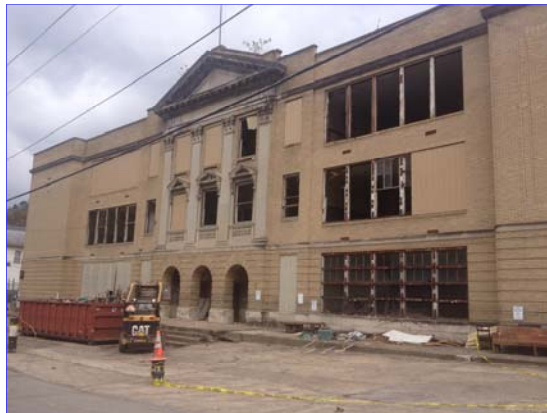
Demolition Underway on the Former Logan High School Building
