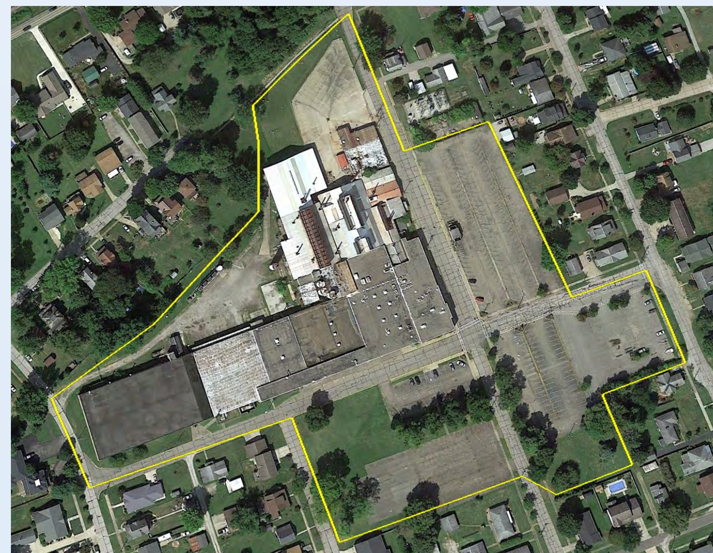
Fenton Art Glass Factory before demolition September, 2015
